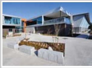
◆ Coquitlam Sports Centre $64 million
